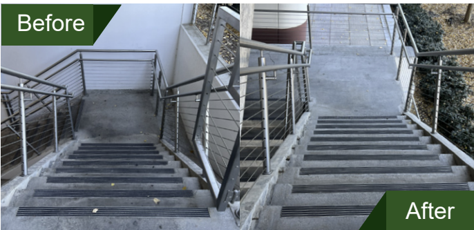
Stairwell Pressure Washing
